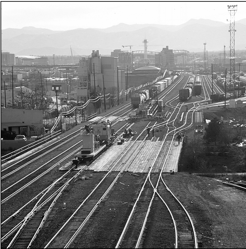
The BNSF's Washington Street underpass is undergoing expansion. BNSF pile driver AX 97502 was in Denver 11/19/02 at the construction site sitting on the main line. Tracks were realigned during underpass construction. Looking from the 38th Street end, left to right tracks are coal two, coal one, the main line and the yard leads (south and north leads with temporary sixth track). – Photo © Chip.
